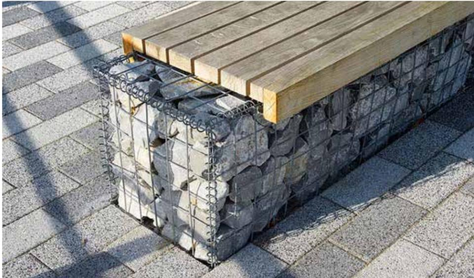
Gabion wall with wood top for seating
