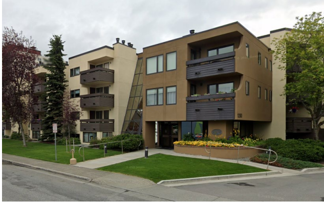
Park Place Condos: A three-story building in South Addition, similar in height to what would be allowed within the TSDO.
