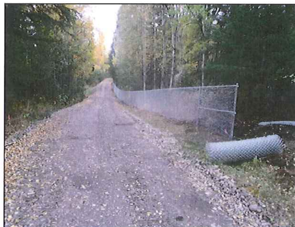
Installation of safety fence near Fish Creek Estuary, looking north.
