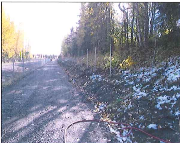
Installation of safety fence near Northern Lights Boulevard, looking south.
