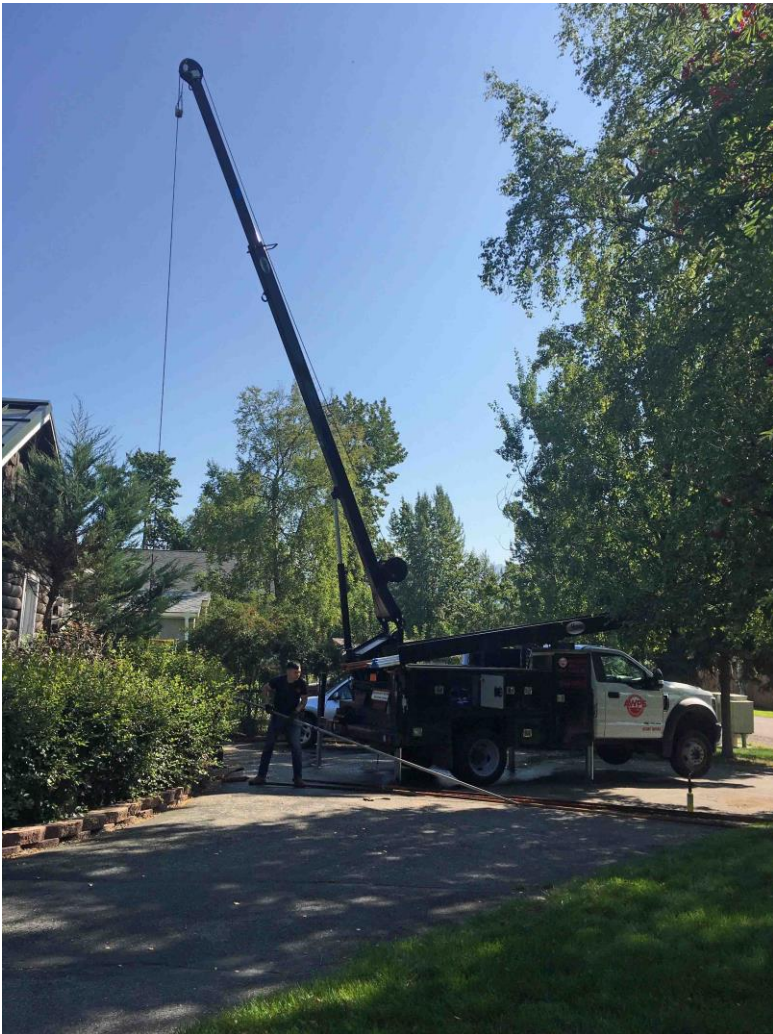
Well Pump and Tubing Replacement Summer 2020 601 Jack Street
