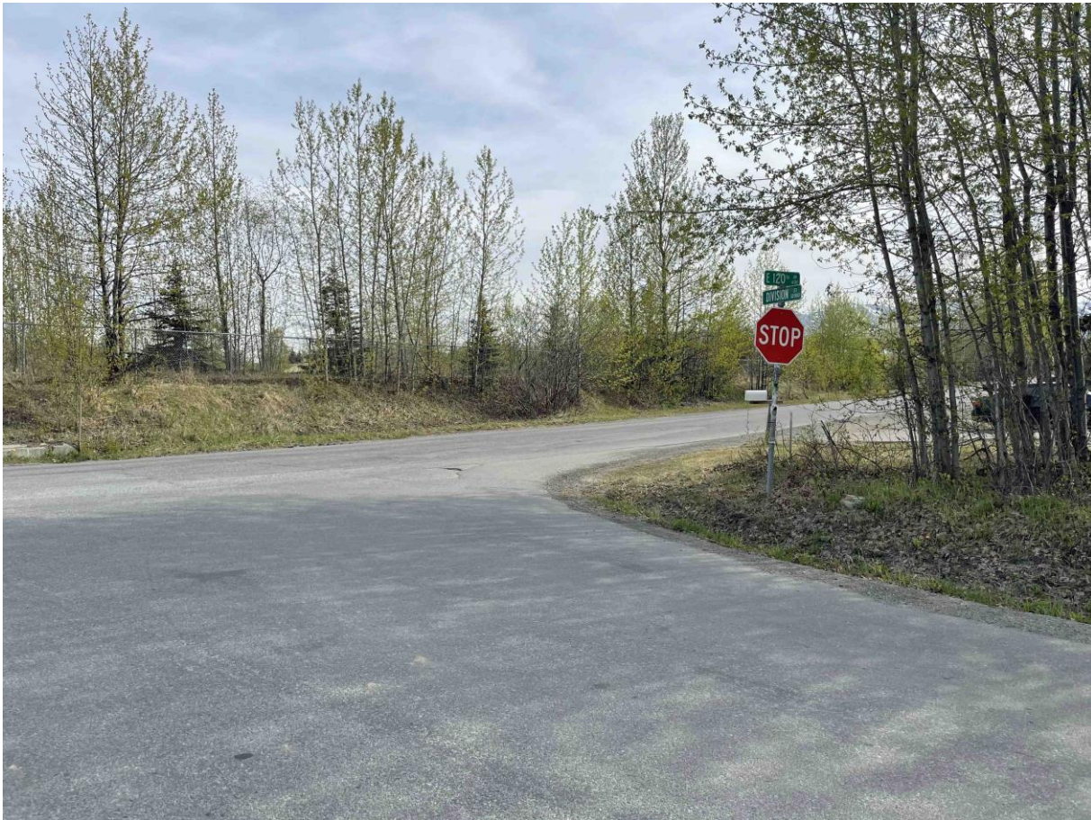
EAST 120 th AVE. @ DIVISION STREET (looking East)
