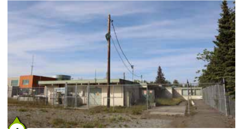
4 View toward site from south
