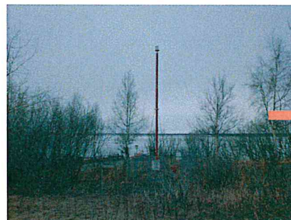
Existing Lighting Tower
