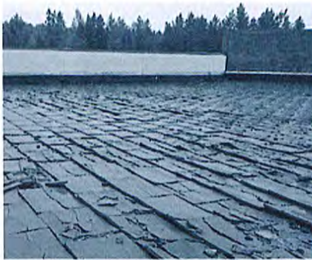
Roof replacement projects are planned for eight buildings.
