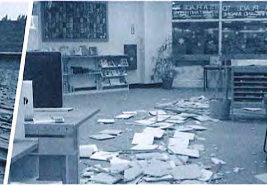
Ceiling tiles litter the West/Romig library after an earthquake.
