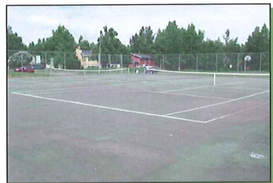
Tennis courts are old and in need of upgrade
