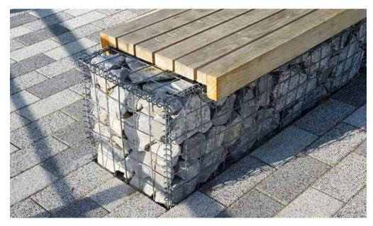
Gabion wall with wood top for seating
