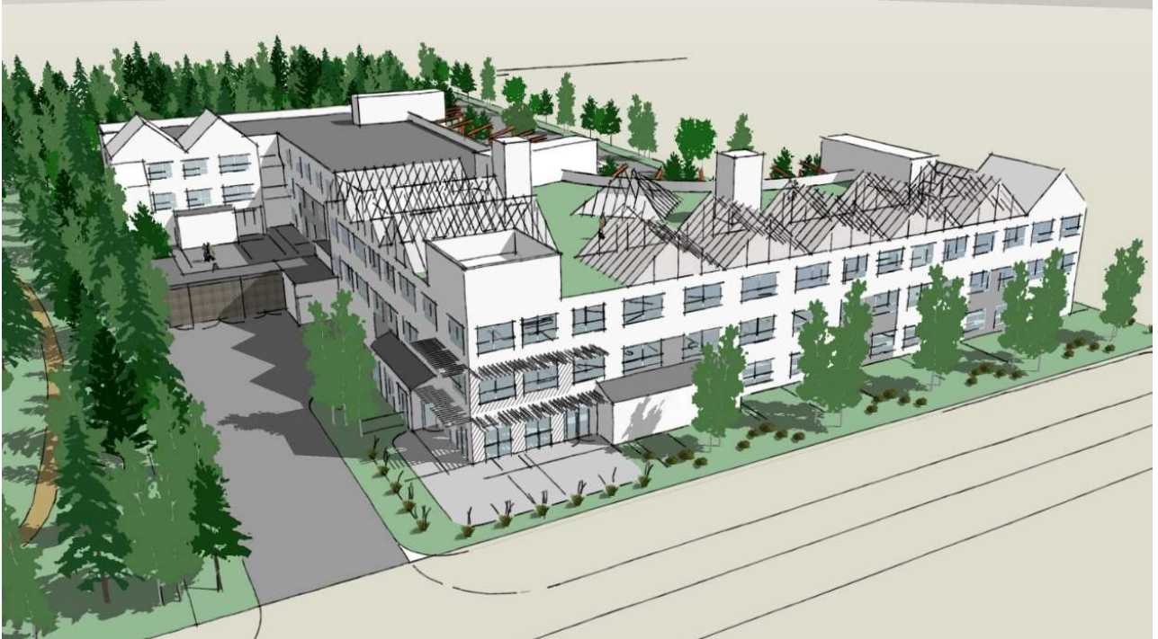
Ariel View of Facility from McLean Road
