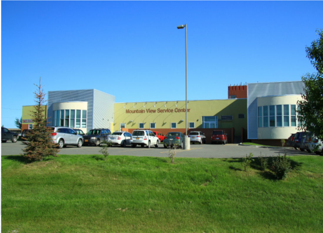
The Mountain View Service Center, formerly the Sadler Warehouse, which was bought and redeveloped by the Anchorage Community Land Trust in 2007 and currently houses eight nonprofit organizations.
