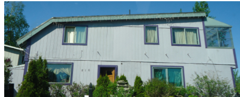
Examples of existing multifamily housing in Mountain View on North Flower Street (at left) and Irwin Street (above).
