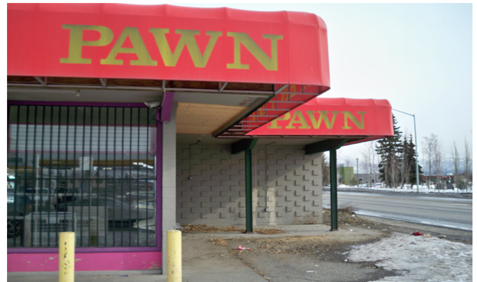
The former Alaska Pawn storefront, on the corner of Price Street and Mountain View Drive. The west side of the building now houses studios for five artists, and the east side will be the new Alaska Regional health clinic.
