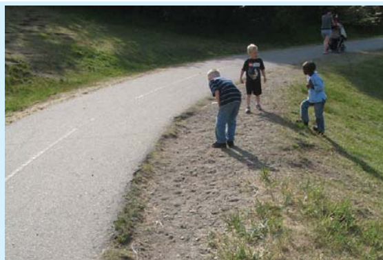
The existing main asphalt path curving around the southern ball field has a very high level of use and its width now exceeds the 2' shoulders.
