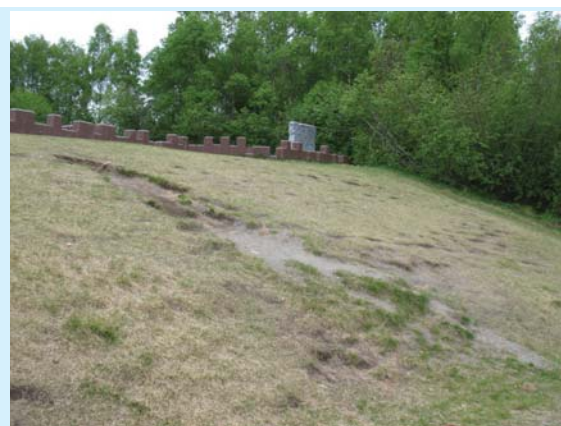
Existing site erosion on the hillside.
