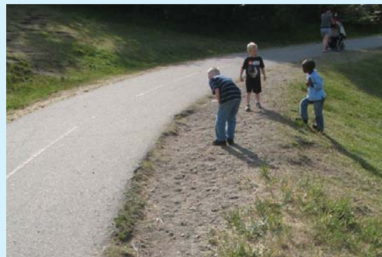
The existing main asphalt path curving around the southern ball field has a very high level of use and its width now exceeds the 2' shoulders.
