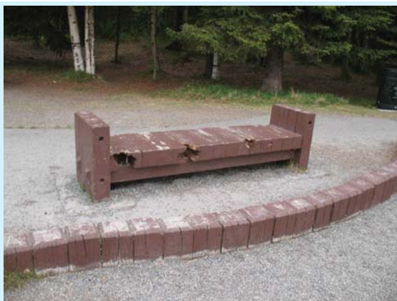
The damage done to this bench in the upper playground area exceeds the Limits of Acceptable Change (LAC) and should be replaced or repaired.
