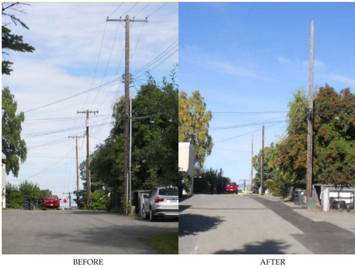
M/N Street Alleys between 7th Avenue and 8th Avenue in Bootlegger's Cove. Poles were left up so communication lines and street lights could remain overhead. Source: ML&P 2019-2023 5 Year Plan.
