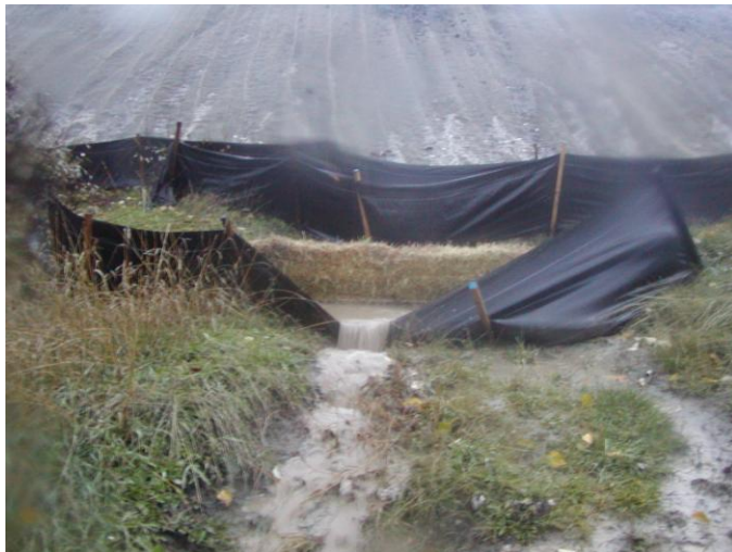
Photo H-1. Flow of turbid water towards South Pond, September 2004.
