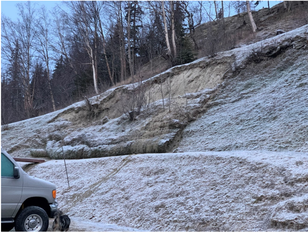
Figure 1. Slope failure on a section of the Rabbit Creek bluff as a result of a property owner clearing and developing steep slopes in violation of Title 21.07.020- (Natural Resource Protection, Section C on steep slope development).
