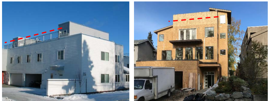
Transparent railing on left and solid parapet at right. Roof access enclosures in both.
