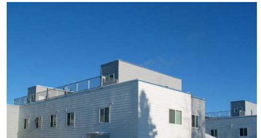
Rooftop access stairwell enclosures and railing on a rooftop deck.
